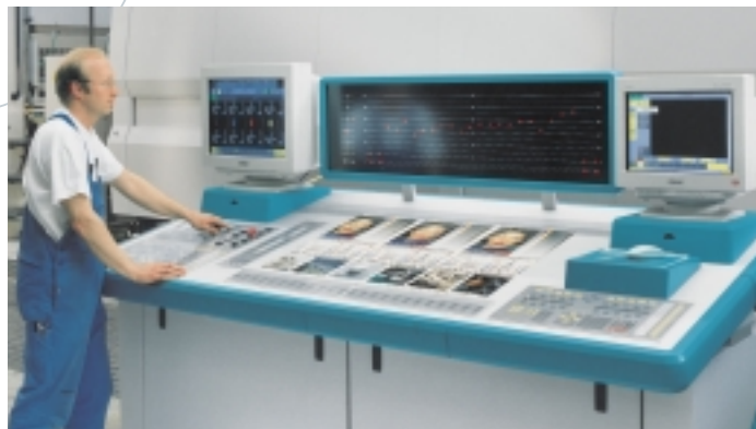
The PECOM central control console, control and monitoring of the entire printing process.
